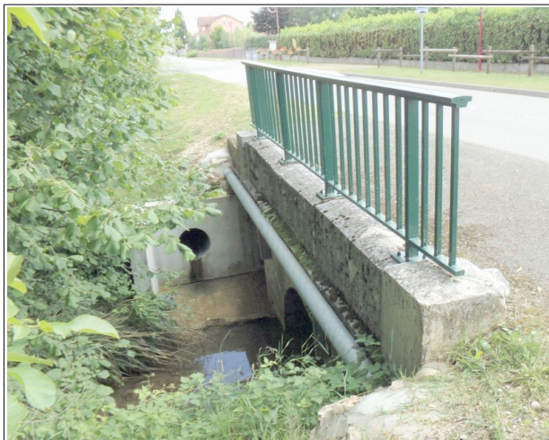
Figure III.63: pont de la RD984
